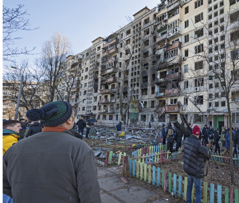
[Damage to an apartment building in Kyiv, an explosion due to a hit by a military shell.] Foto: iStock.
